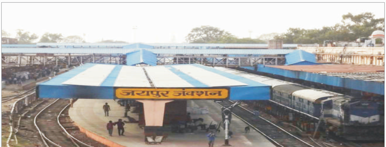
Solar rooftop power plant at Jaipur Railway Station
