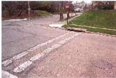
Intersection Jiggle Bumps. (Dayton, OH)
