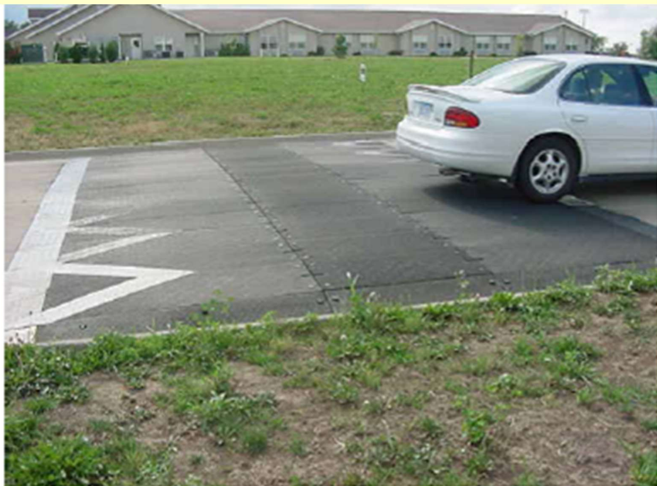
Figure 18. 18-Foot Temporary 30 mph Speed Table
