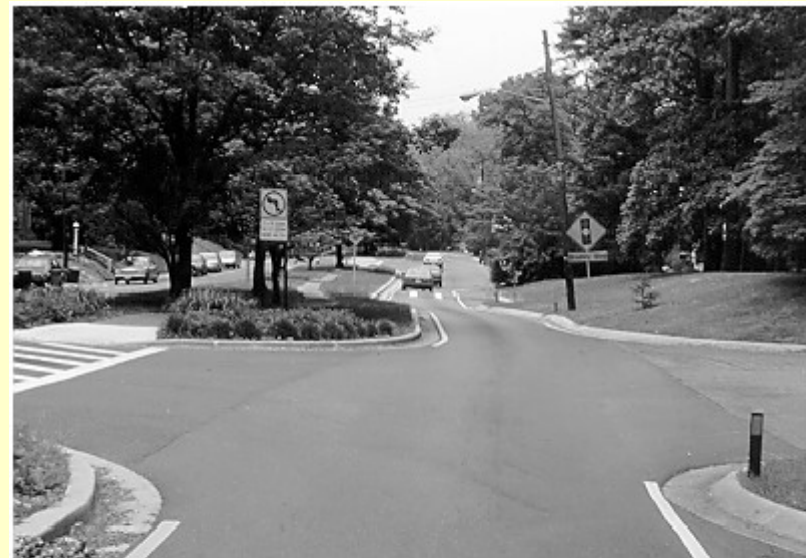
Figure 5.14. Chicanes/22-foot Speed Tables. (Huntington Pkwy.—Montgomery County, MD)
