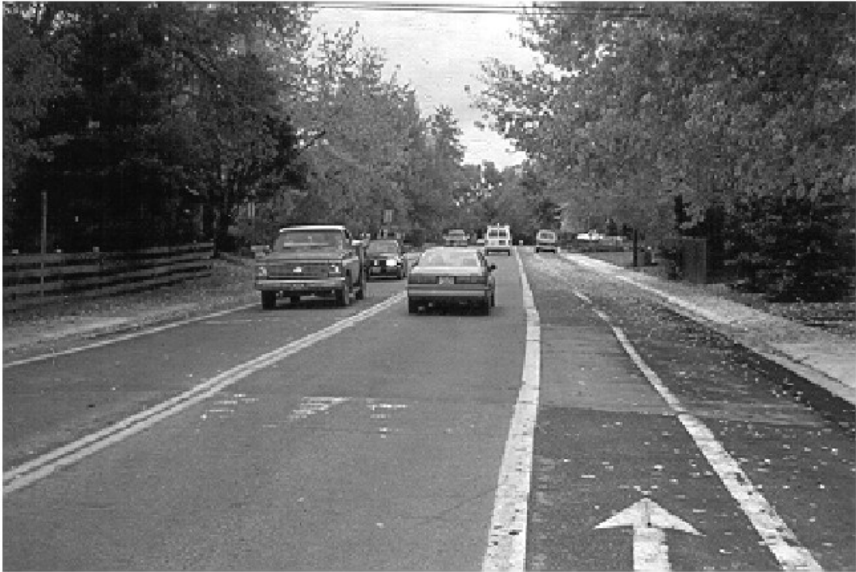
Figure 7.8. Former Speed Table Location on Edgewood Drive.
