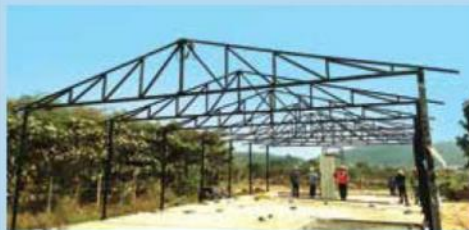
Tubular Steel Structure
