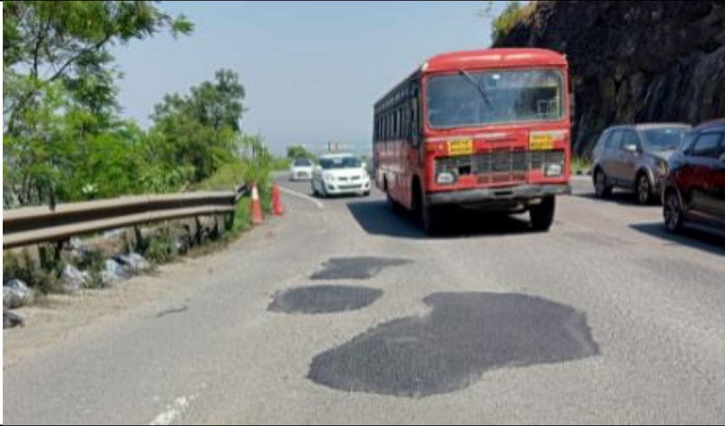
Potholes repairing at Ch 774 to 780 RHS Ghat Section
