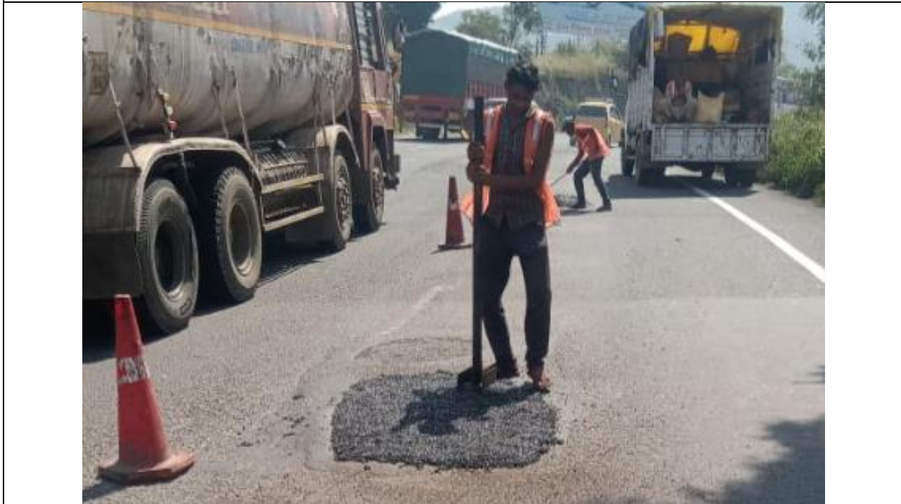
Pot hole Repairing using Cold mix at Ch.-780+00 RHS MCW
