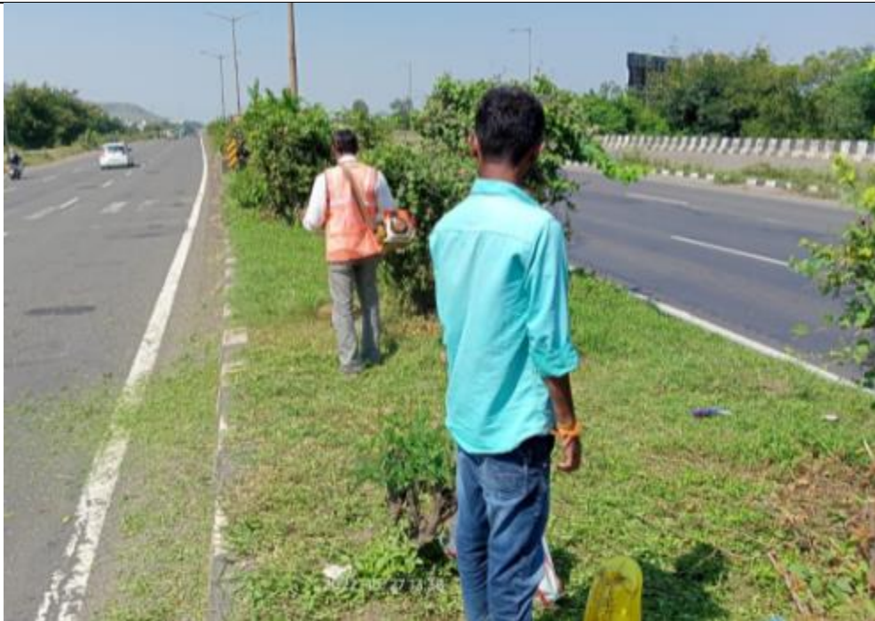
Median grass cutting is in progress at Ch 743
