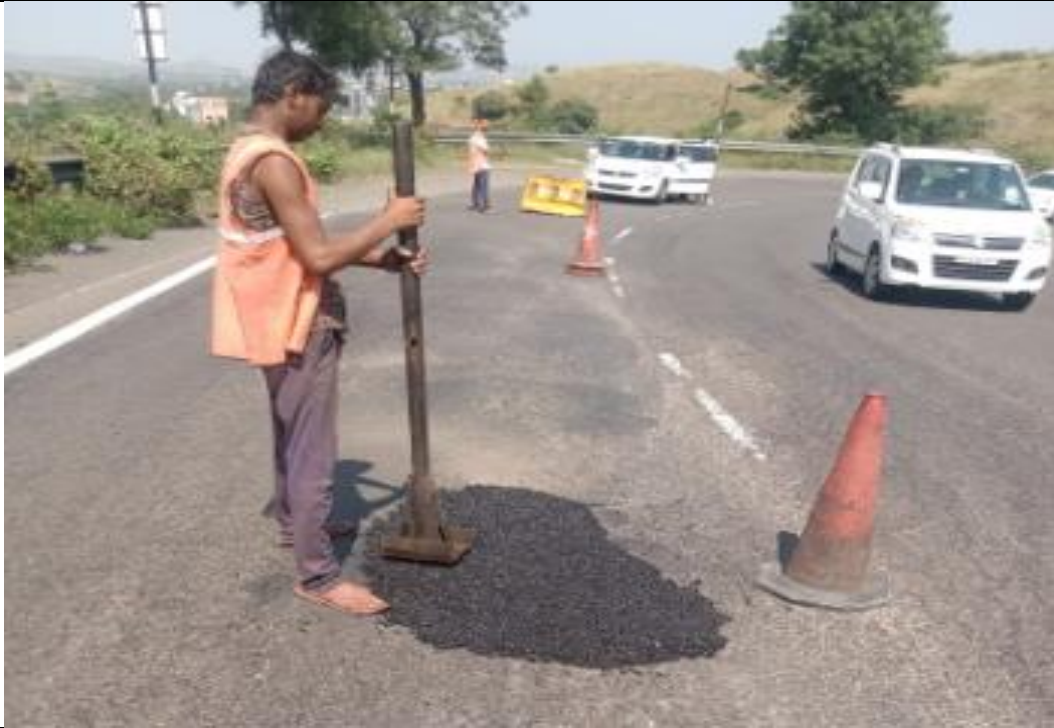
Pot hole Repairing using Cold Mix at Ch. 780+050 RHS MCW
