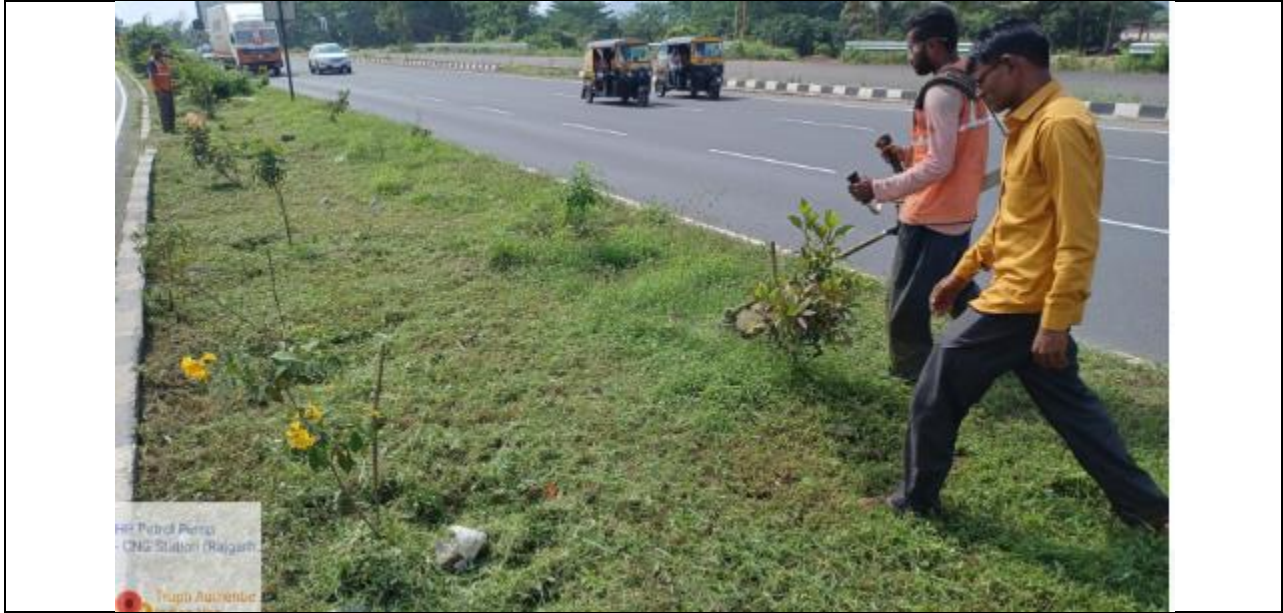
Ch.816+400 to Ch.817+000 Median Grass Cutting work
