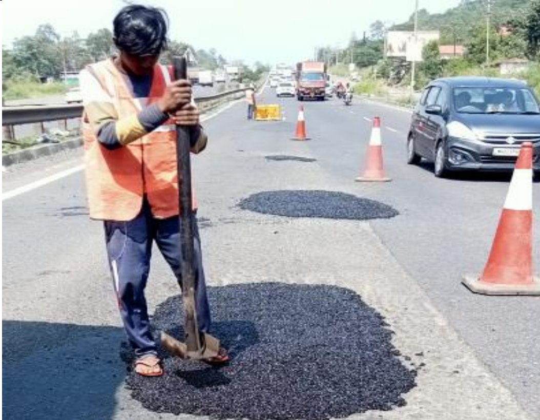
Pot hole Repairing using Cold Mix at Ch. 810+330
