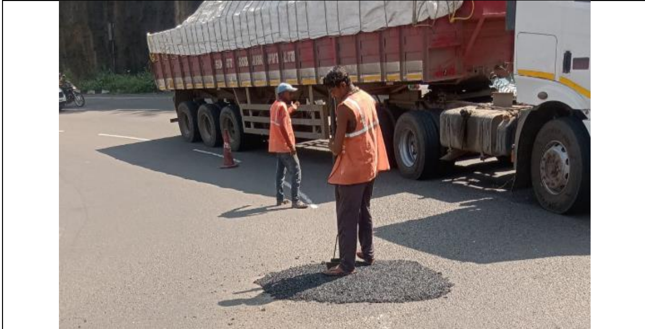
Pot hole Repairing using Cold mix at Ch. 775+750 RHS MCW
