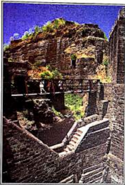
Rock cut well seen inside Daulatabad fort is 16m wide & 22m deep
