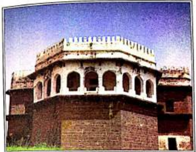
Bastion, an octagonal palace having twelve arches, built during the reign of Shahajahan.
