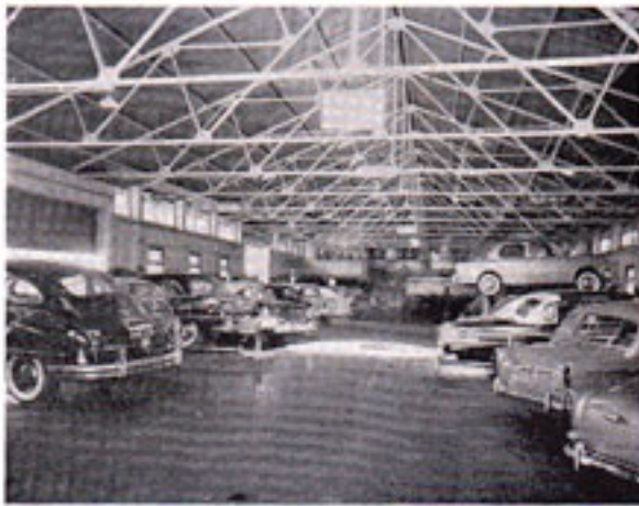
Reception and light repair section at Tardeo Service Station.
